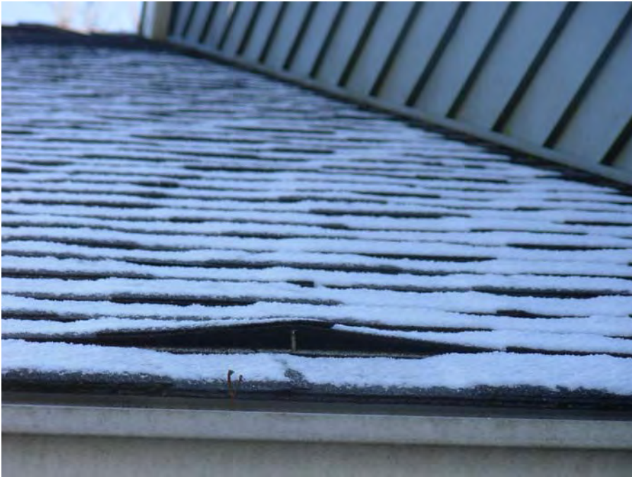
5. Spot lifting and nail popping under roofing shingles
