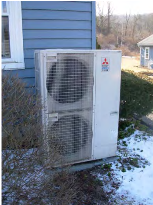
9. Exterior condenser-compressor for cmnty. bldg. heat pump HVAC
