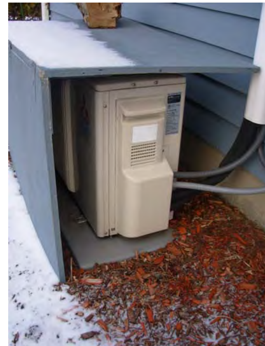
16. Typical unit heat pump HVAC system, exterior condenser-compressor
