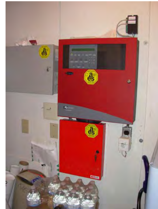
10. Fire detection and ECAS monitoring system
