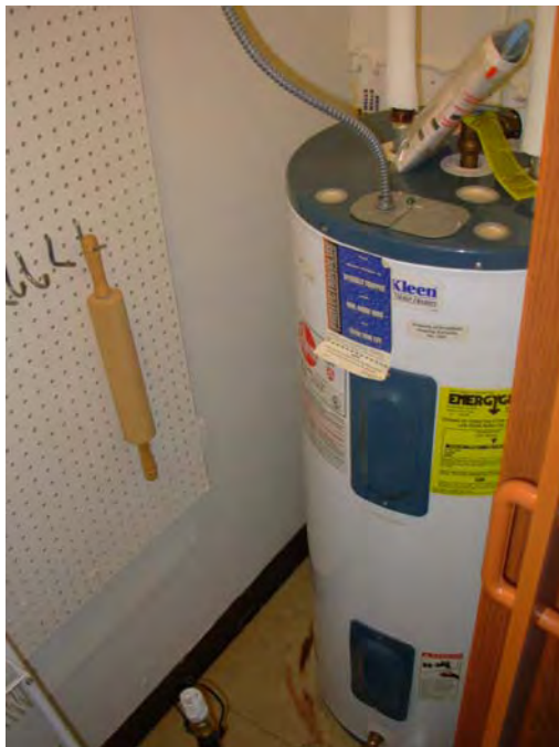
15. Typical unit DHW tanks, electric
